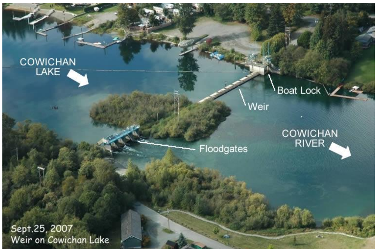
Photo 6-1: Existing Weir (Source: Cowichan Watershed Board)
